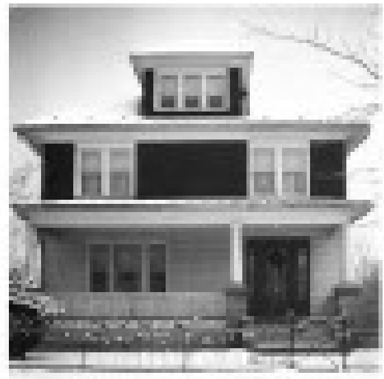
The Belzoni family home at 101 East Eighth Street, Wyoming, PA
