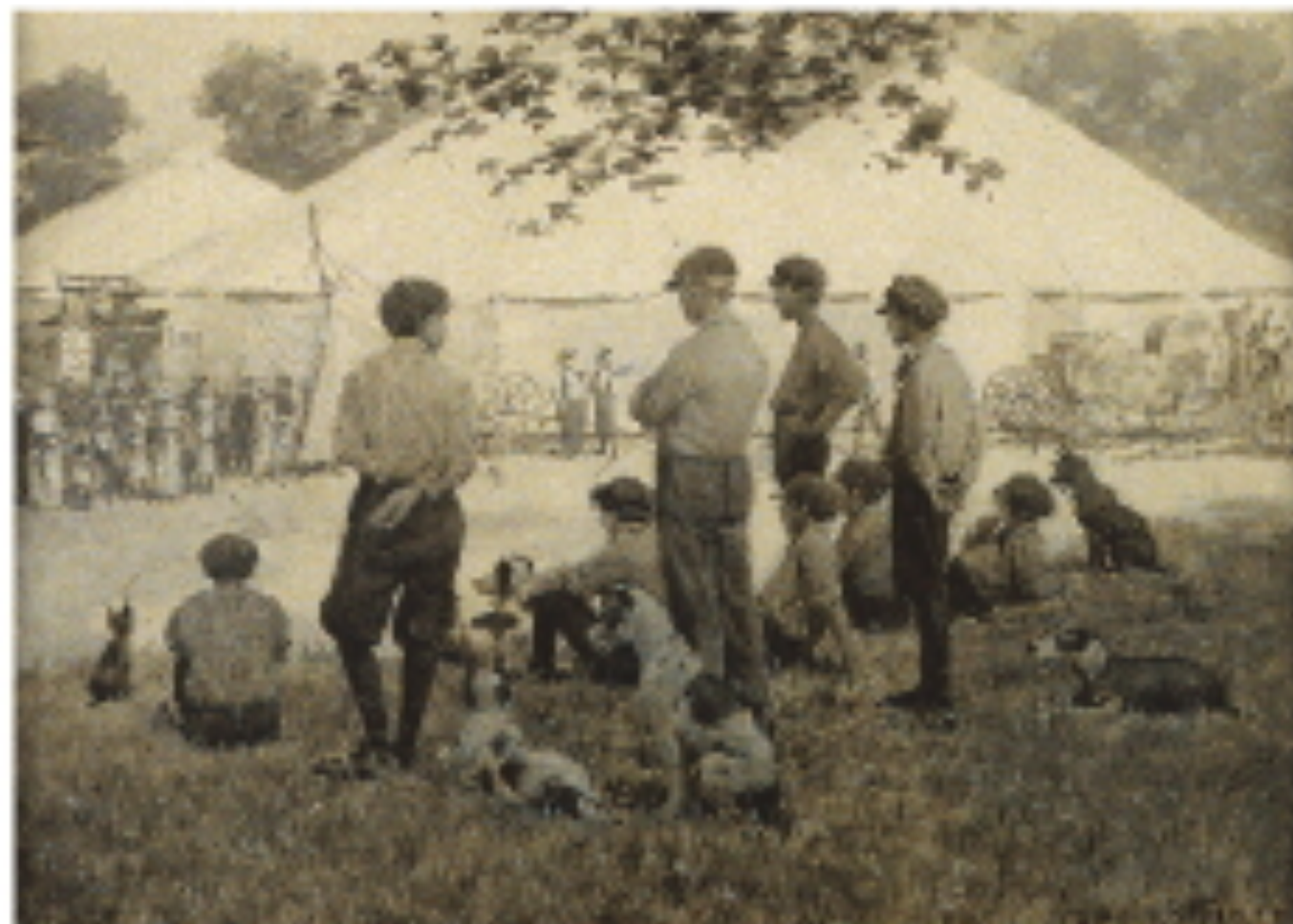
Digital Restoration. Milwaukee on board. Photo courtesy of Illustration House, WI
